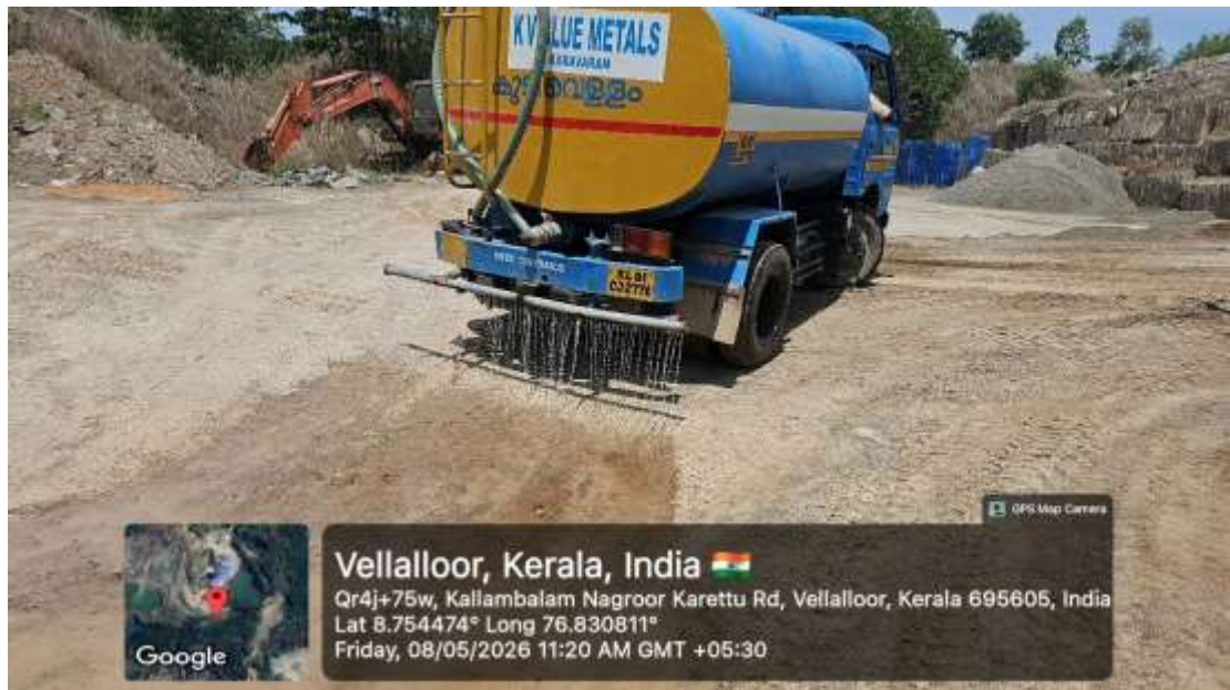
Figure 6 : Photograph Showing Dust Suppression Measures Using Water Tanker Lorries
